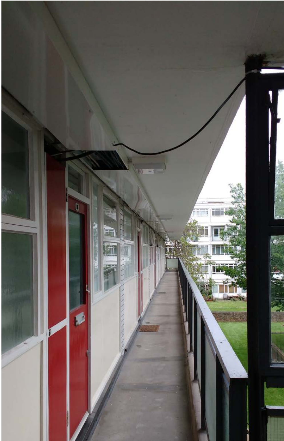
View of underside of walkway
